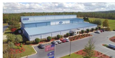
Gaston, South Carolina Manufacturing Plant
